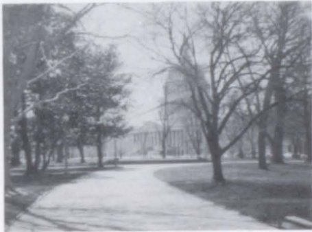
The Capitol Building
